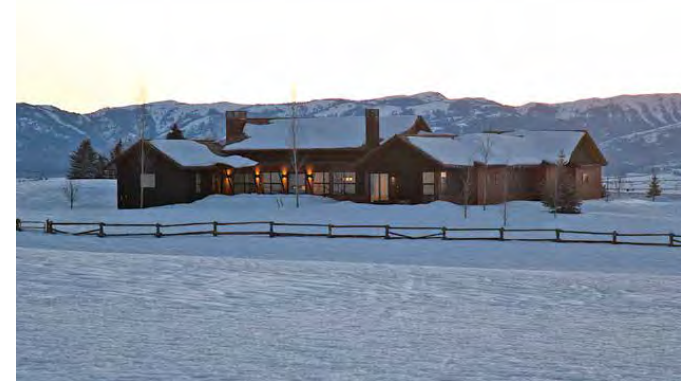
The home's low profile and H shape make it inherently stable against gale-force winds. This geometry, combined with its exterior rain-wall system and triple-pane windows, creates an industrial-strength and deadpan-quiet home even under the most extreme weather conditions.
