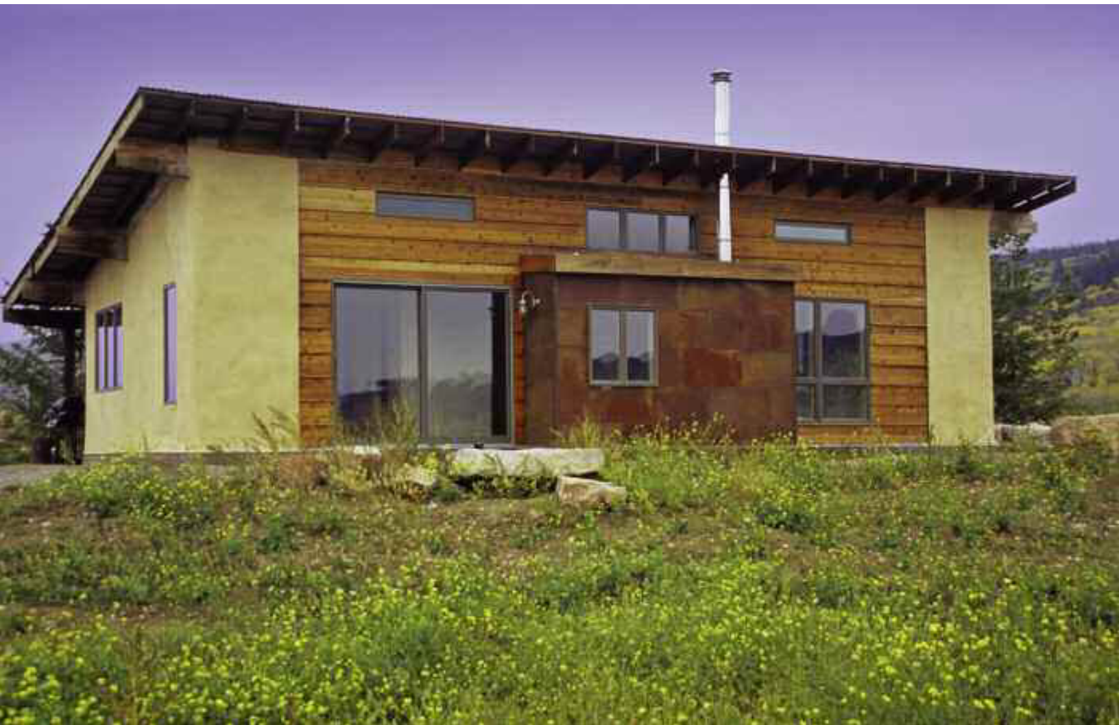
The simple shed roof is raised above the south-facing wall to admit generous passive solar heat and light. The projecting metal-clad enclosure houses a couch and stove.
